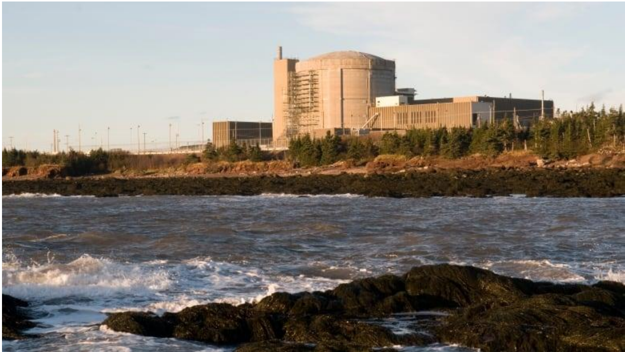
Figure 1. Point Lepreau CANDU Six 705 megawatt reactor in New Brunswick Canada in 2020, then running above 90% capacity. It was commissioned in 1983 and refurbished in 2012. Although renovation was supposed to begin in 2008 the whole process was itself delayed by operating problems so that renovation actually began in 2011 and took a year. Cost over-runs and insurance problems delayed its re-start. Apart from well-known environmental sustainability questions, Point Lepreau is a text book-case on the difficulty of successfully operating a reactor of this size, triggering both planning and financial issues. The high cost of insurance for the renovated reactor was confidential, adding to the cost of a unit of electricity from Point Lepreau. As the cost was difficult to measure, it is thus difficult to compare it with other reactors, particularly with respect to its contribution to climate change. The original Point Lepreau reactor was built long after the early CANDU reactors were installed in Ontario, India, Pakistan, Korea and Argentina. (NB Power, Point Lepreau nuclear generating station , photograph published Jan 28, 2021 by CBC news, https://www.cbc.ca/news/canada/new-brunswick/lepreau-nbpower-nuclear-plant-1.5890989 . Image used with permission. Rights belong with NB Power.)
