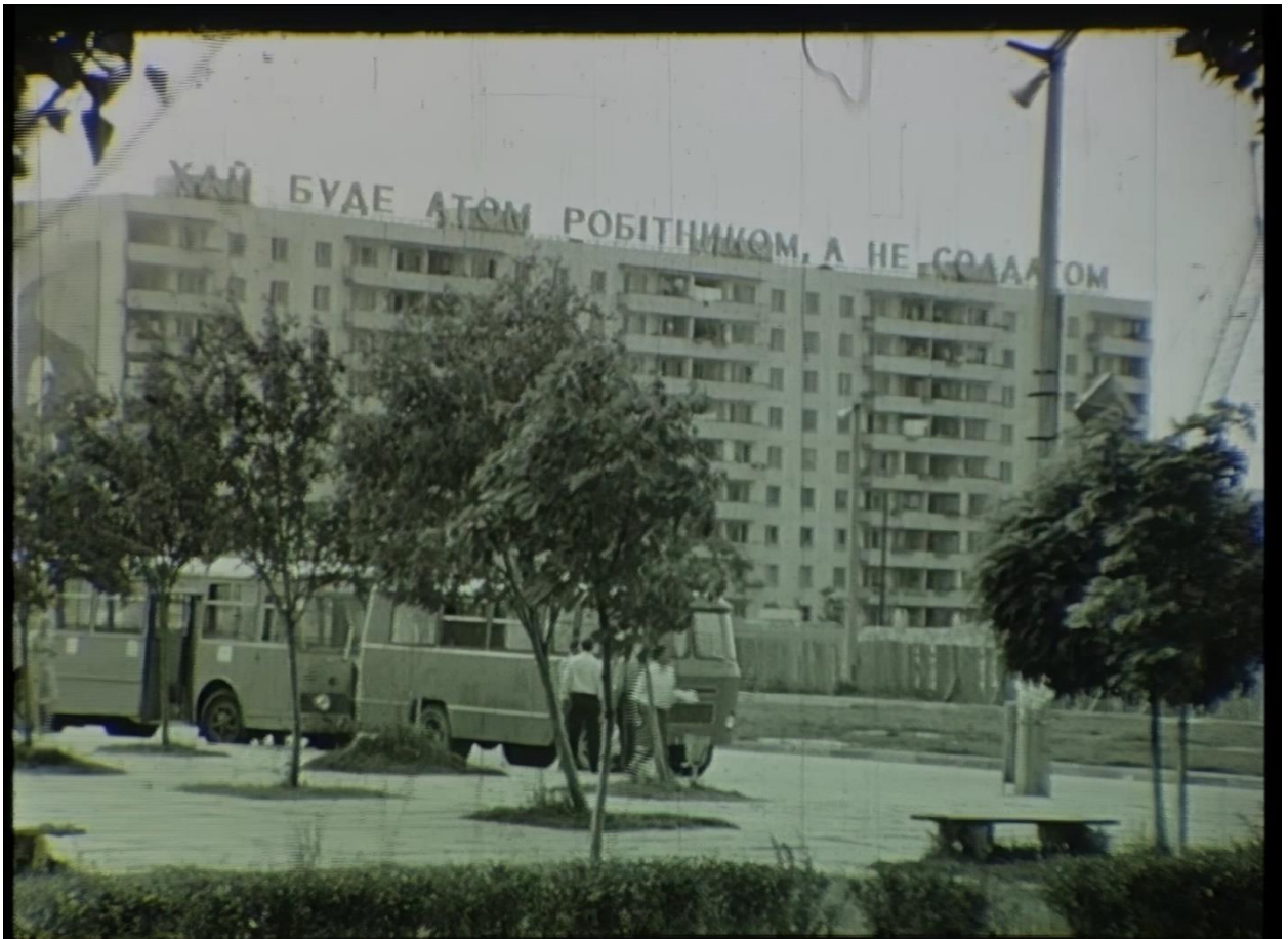
Figure 13. An apartment building #3 on Sergeant Lazarev Street in Prip'yat featuring a celebratory slogan typical for the Soviet atomic cities, “Let the atom be a worker, not a soldier,” that supported and reinforced the ideological narrative about “peaceful atom.” Although its scale cannot be fully assessed and understood today, I am reading the bodies of the subjects of territory (human and non-human) as a collective body-archive where epigenetic transformation occurs. This mark is a direct imprint of the state techno-politics and its information policy on risk communication (or rather, a lack thereof) made the subjects connected, subscribed, and subordinated to the contaminated territory – biopolitically. The promotional slogan proudly installed on the top of one of the highest buildings was seen by many citizens as a reversal of the truth, which paradoxically revealed the impossibility to hide it and served as its expression in a
