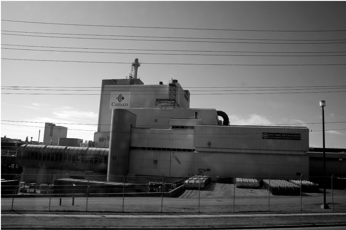
Figure 9. The oldest refinery of uranium in the world, Cameco, once known as Eldorado Mining and Refining Ltd., is located on the outskirts of the Town of Port Hope in Ontario, Canada. The facility processed and refined weapons-grade uranium, and in this process produced copious amounts of low-level waste that contaminated the local area. It is these activities that have been at the center of radioactive public health controversy in Port Hope, including controversies of transparency around the provision and access to data and studies. (Photographer Robert Taylor, Cameco Nuclear, Port Hope, Ontario_4715, June 20, 2011, https://www.flickr.com/photos/bobolink/5857844634/in/photostream/ . Used under a CC BY 2.0 Generic license.)
