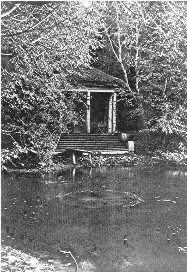
D. Efimov. The Little House in Tsarskoe Selo in Memory of Grand Duchess Aleksandra Nikolaevna . 1845. Wood construction. (Vil'chkovskii, Tsarskoe Selo , facing p. 190)
